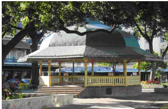
Restoration of the Alamo Plaza Bandstand
